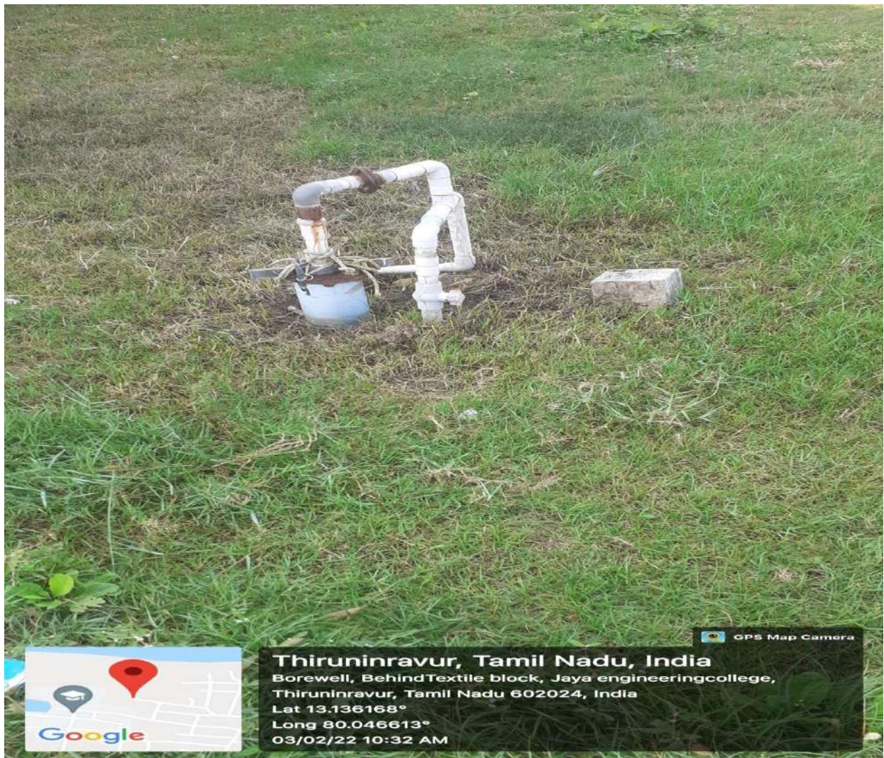
Bore well in textile back side, Submersible motor Capacity : 3 Hp
